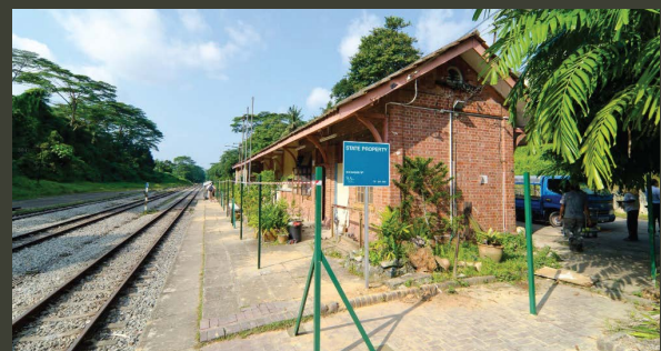
Bukit Timah Railway Station
