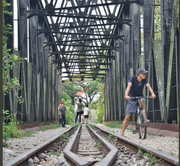
The popular steel truss bridge along Bukit Timah Road
